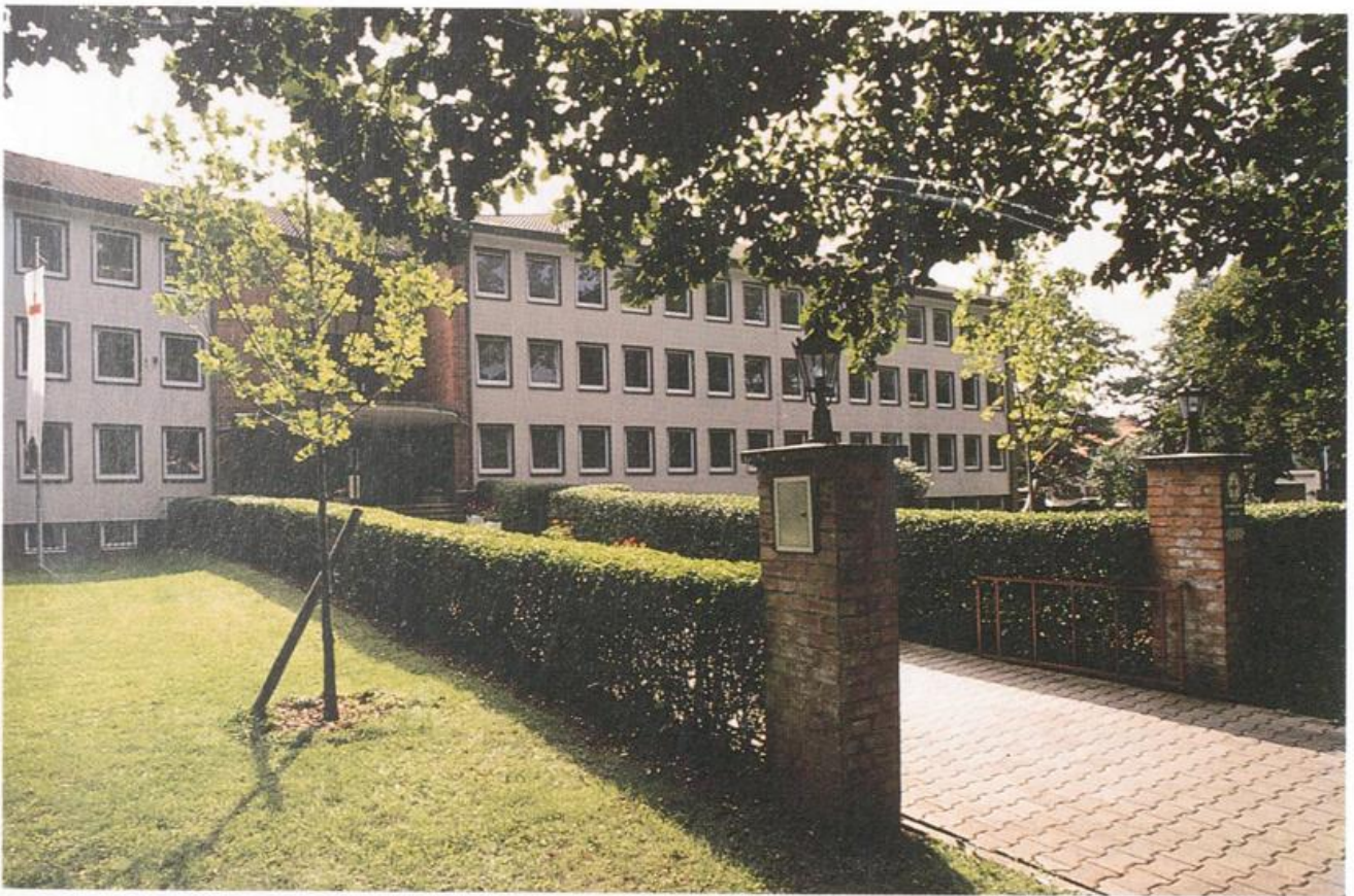
The Main Building of the International Tracing Service in the Grosse Allee
